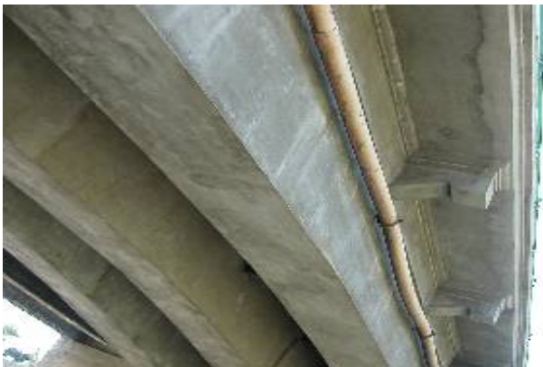
Reparation with thixotropic mortar
