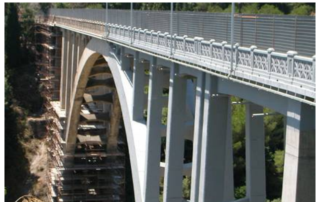
Reparation with thixotropic mortar
