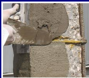
Reparation with thixotropic mortar
