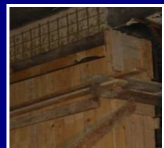
Pilars (increase section)
